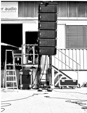
Fig. 8: Picture of the measurement setup: Nexo GEO S12 line-source array with pressure zone microphones on the floor.
