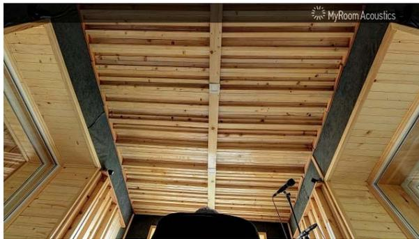
Figure 9 Ceiling treatment of first Control Room designed following new principle.
